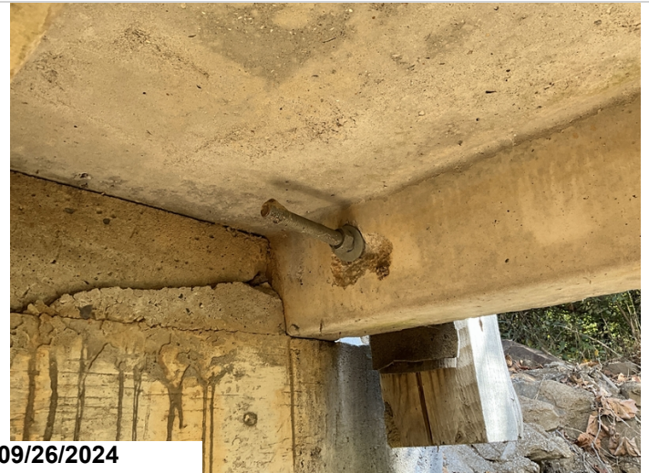
Span 1, bent 1, unit 1 left leg has spalling at lag bolt. CS3
