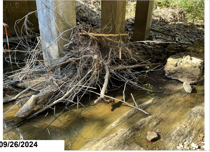
Span 2, bent 3, has drift build up in between the columns.
