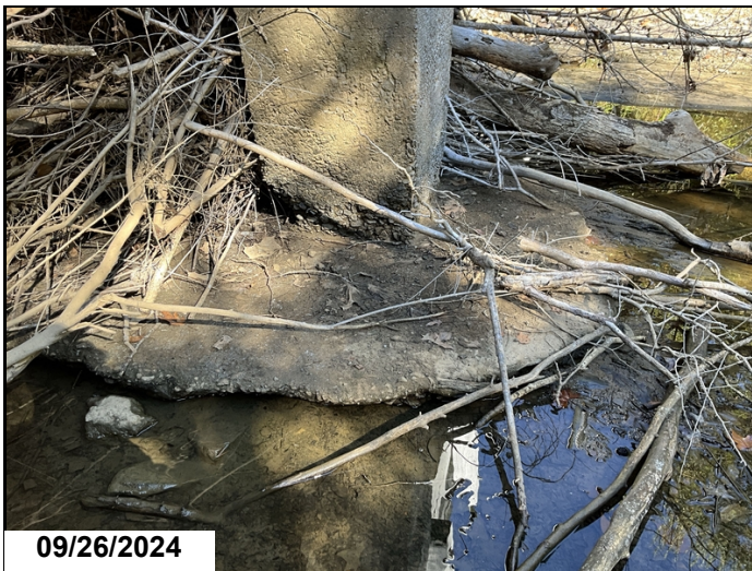
Span 3, bent 3, column 1, has section loss.
