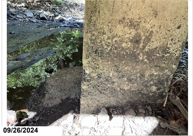
Span 1, bent 2, column 2, has spalling. CS3
