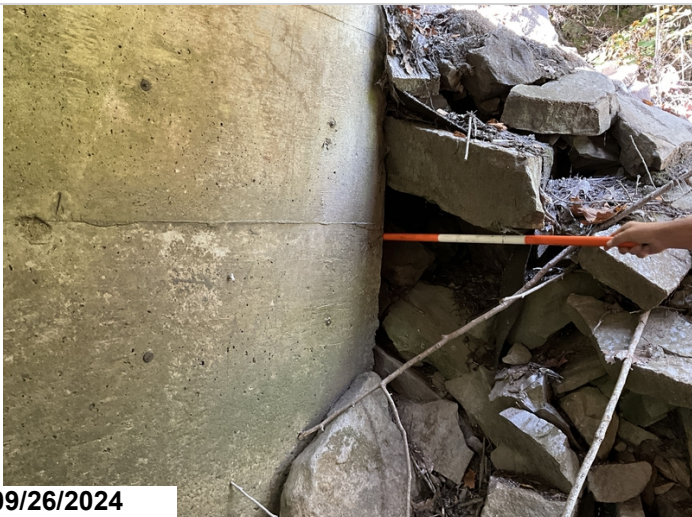
Span 3, bent 4, right side has erosion approximately 1'.
