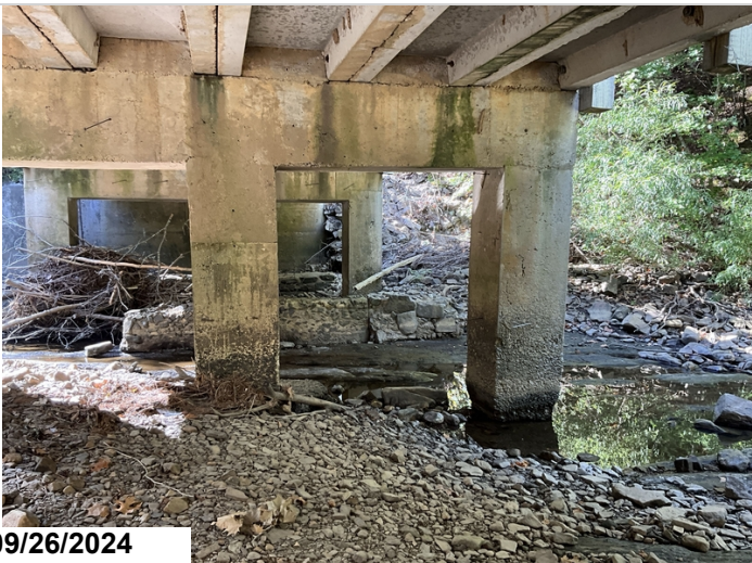
Span 1, bent 2, column 3, has concrete deterioration. CS3
