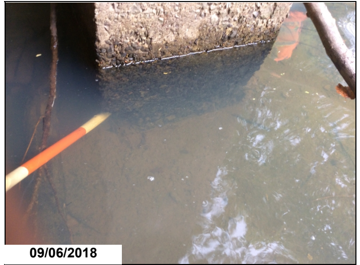
Bent # 3 Lt column concrete deterioration with section loss.
