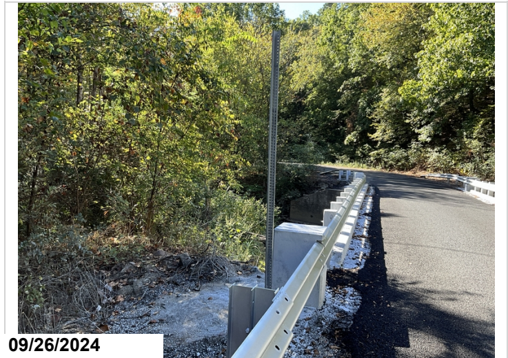
Span 1, bent 1, left side approach is missing flare panel.
