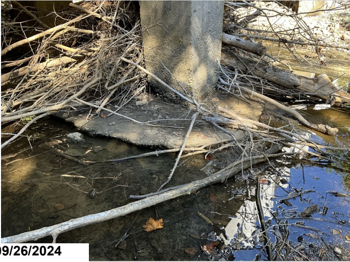
Span 3, bent 3, column 1, has spalling. CS3
