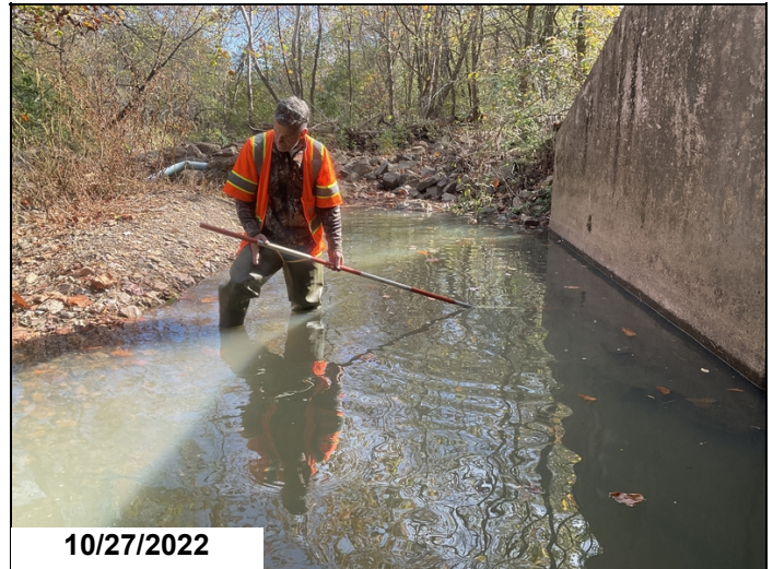
The Southeast wing wall has a non uniform footing with voids that penetrate approximately 12" under the edge of the footing. Voids do not reach the face of the wing wall during this inspection.
