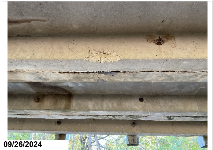
Span 3, bent 3, unit 3 left leg has spalling. CS2
