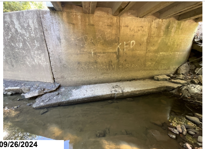
Span 3, bent 4, footing is exposed.
