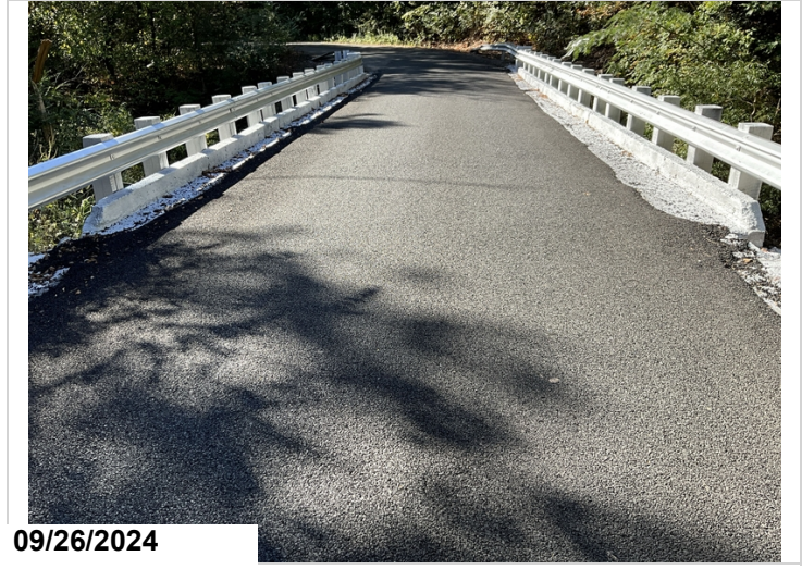
Deck has new asphalt wearing surface . 3"
