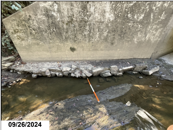
Span 3, bent 4, left side wing wall undermining.
