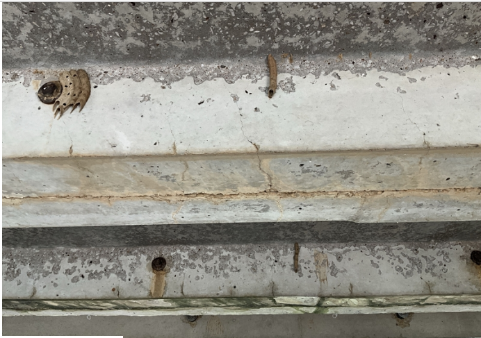
Span 1, bent 1, unit 4, right leg has flexure cracking. CS2
