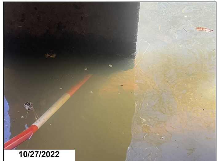
Bent 3, column 1-Concrete section loss at base of column
